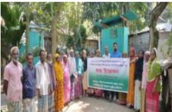
Semi-paved Latrine Installation for ultra-poor family
